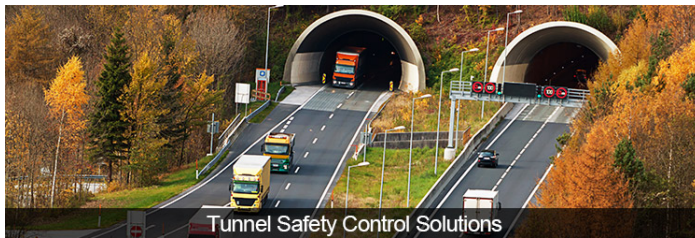
Tunnel Safety Control Solutions
